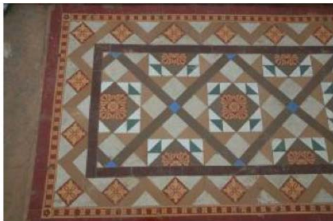
a: Floor tiles of porch in FML
