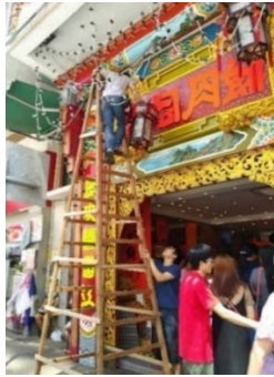
Fig 12 Unloading lanterns, part of the festive pavilions, at the day when typhoon was issuing. Wooden ladder was sitting in front of the store, covering the pavement. Photographed by Nicole Lee.
