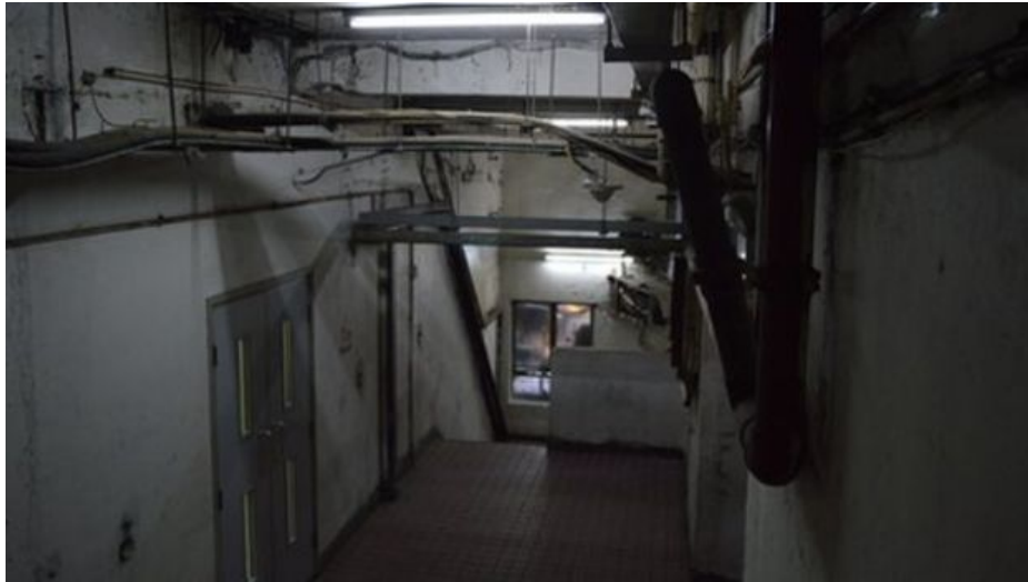
Isolated corridors and stairwells connect different parts of the building complex
